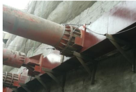
Fig. 11 Implementation Effect Diagram 1 of the Steel Hanging Plate for Improving the Cantilever Bracket
