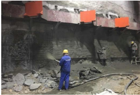
Fig. 11 Implementation Effect Diagram 1 of the Steel Hanging Plate for Improving the Cantilever Bracket
