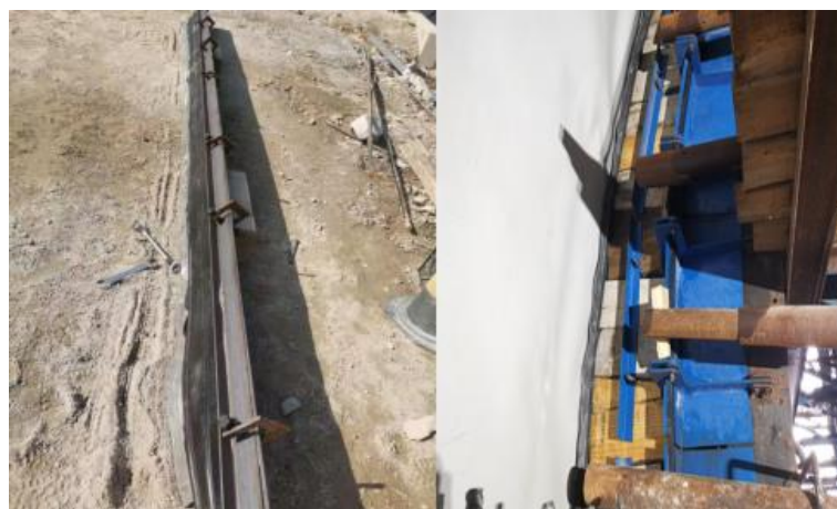
(a) 纵向止水带定位夹具 (b) 钢端模模块 (a) Longitudinal Waterstop Positioning Fixture (b) Steel End Formwork Module
